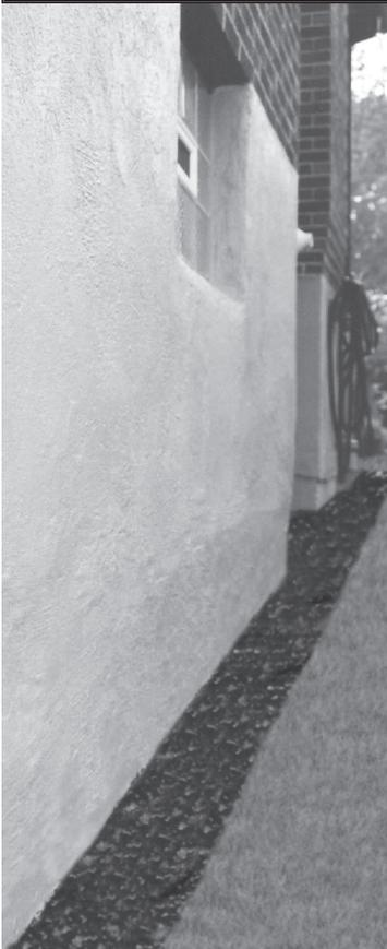
The majority of basement wetness problems stem from improper drainage or grading around the foundation
